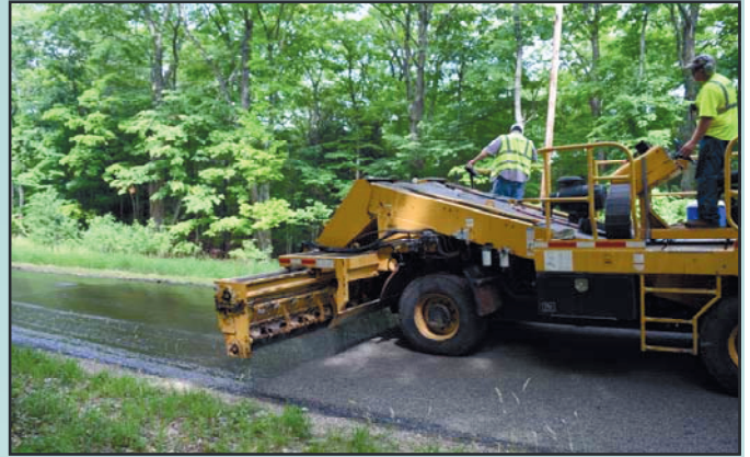
Aggregate Spreader during the chip sealing process
