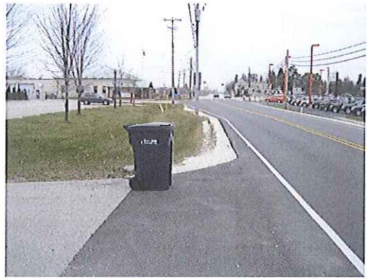
Location – The cart is within 3' of the edge of pavement.
